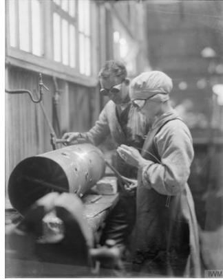
Fig. 12. A member of Queen Mary's Army Auxiliary Corps (QMAAC) acetylene welding at a Royal Air Force engine repair shop at Pont de l'Arche, France, in 1919; Olive Edis; “Q8117”; *The Imperial War Museum*; [iwm.org.uk](http://iwm.org.uk); 1919; Web; 14 Jan. 2016.
